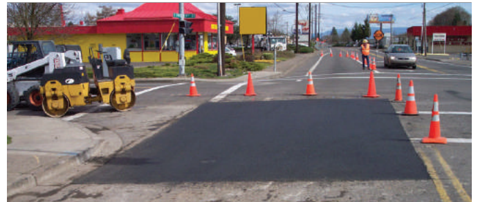
ROAD RECLAMATION / REPAIR
