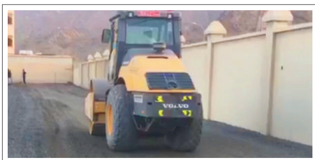
STEP 5 COMPACTING THE WAY
